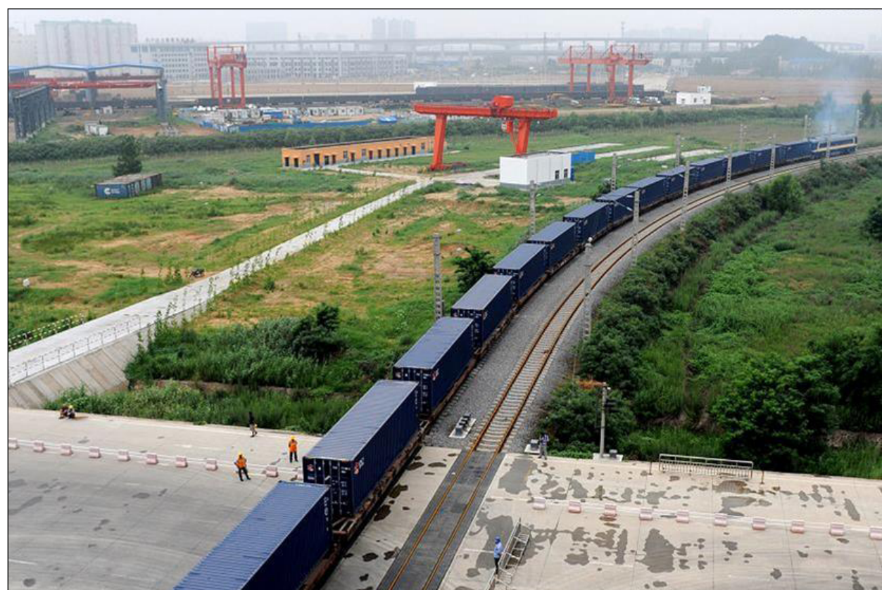
Photo taken on July 18, 2013 shows the first direct cargo train leaving from Zhengzhou to Europe at the railway container center in Zhengzhou, capital of Central China's Henan Province.
